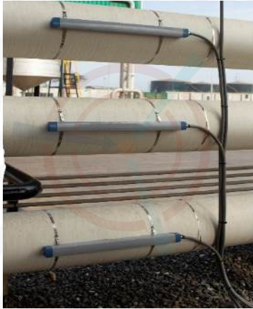
SML Ultrasonic Flowmeters on Depot Pipes
