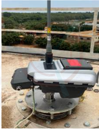
SML Automatic Tank Gauging System(ATGs)
